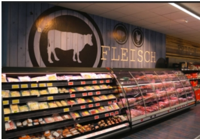
Figure 1: A cabinet connected to the chilled waterloop
