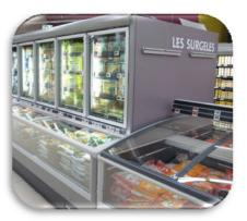
All the low temperature cabinet doors are closed in the Super U to avoid energy losses.
