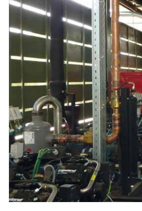
efficiency, emissions reduction and refrigeration performance. Honeywell's Solstice N13, selected for the MT system, is a new generation HFO refrigerant blend that is a non-flammable, non-ozone depleting replacement for R-134a, with 60% lower Global Warming Potential (GWP).
